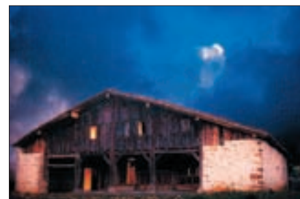
Figure 1: Front view of the Igartubeiti farmhouse
